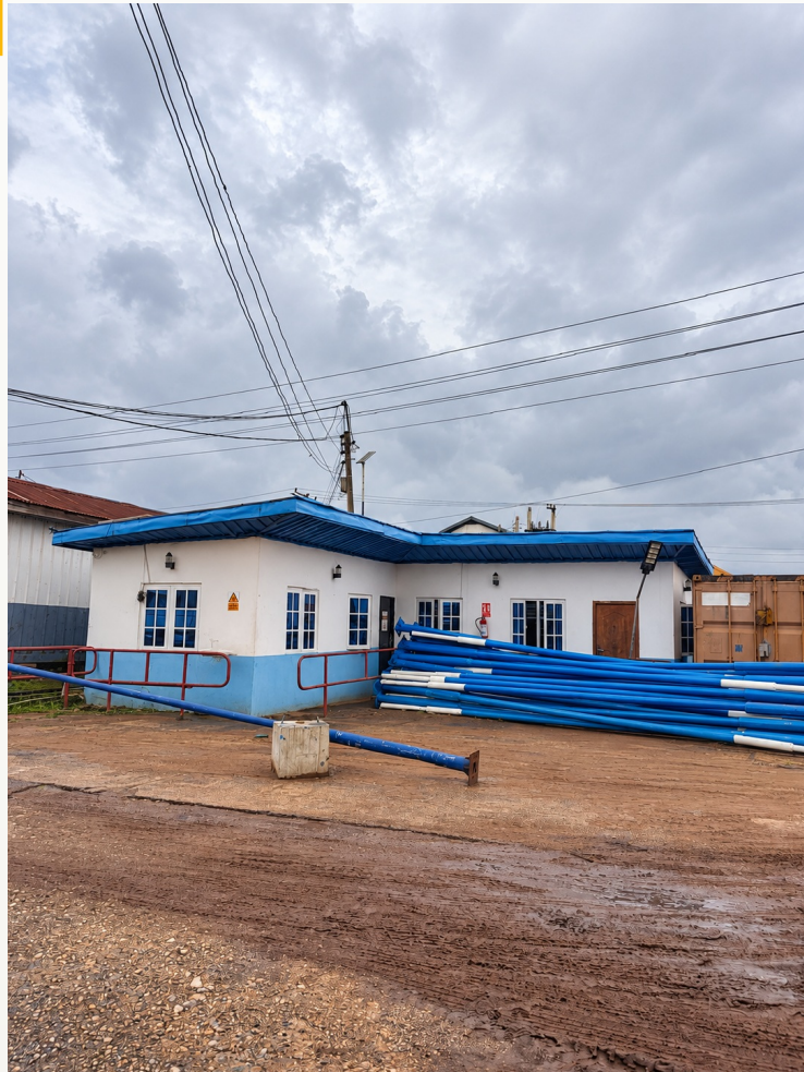
Field support facilities
