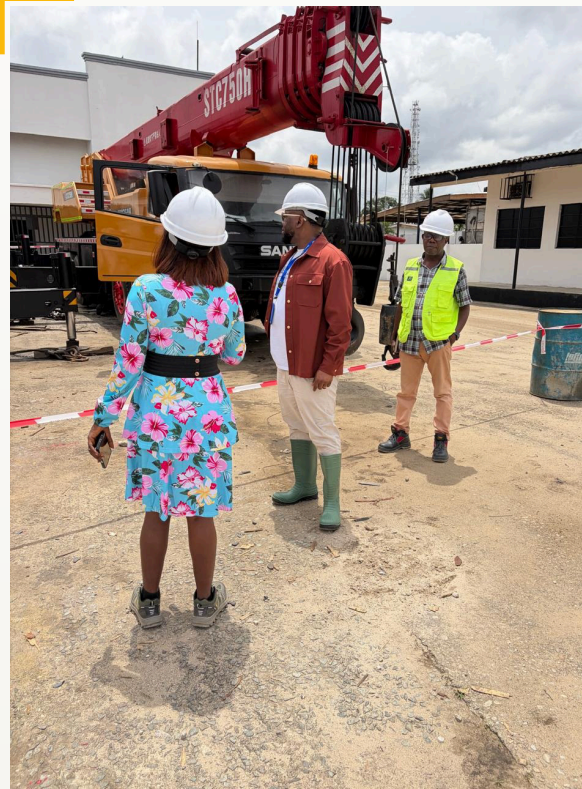
Equipment and lifting
